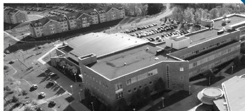
Pictured: The College's three new residence halls (left background), the Whitney Applied Technology Center (center) and the Gordon Student Center (right background).
